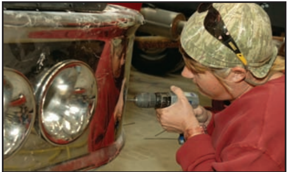
Patricia Roe, an electrician with Ferrara, drills holes to install a warning lamp on the bumper of an apparatus under construction. Ferrara builds units on a wide variety of cabs and chassis, including its own line.
